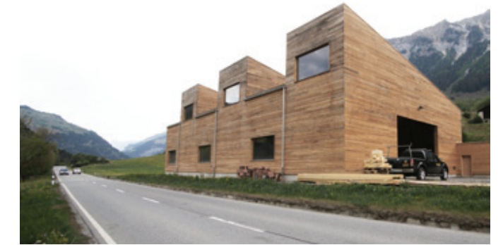
▲ Mani Holzbau Iseppi/Kurath's participatory approach to the Mani Holzbau woodworks yard resulted in a simple yet elegant structure
